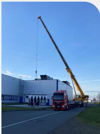
Figure 7: Installation of the heat pump system in Germany.
